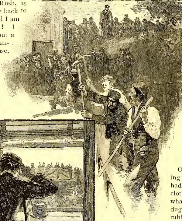
"A LINE OF MEN DEMOLISHING THE DAM."
