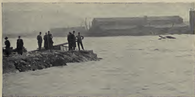
Franklin Bridge, 6.30 P.M., Showing Total Collapse
