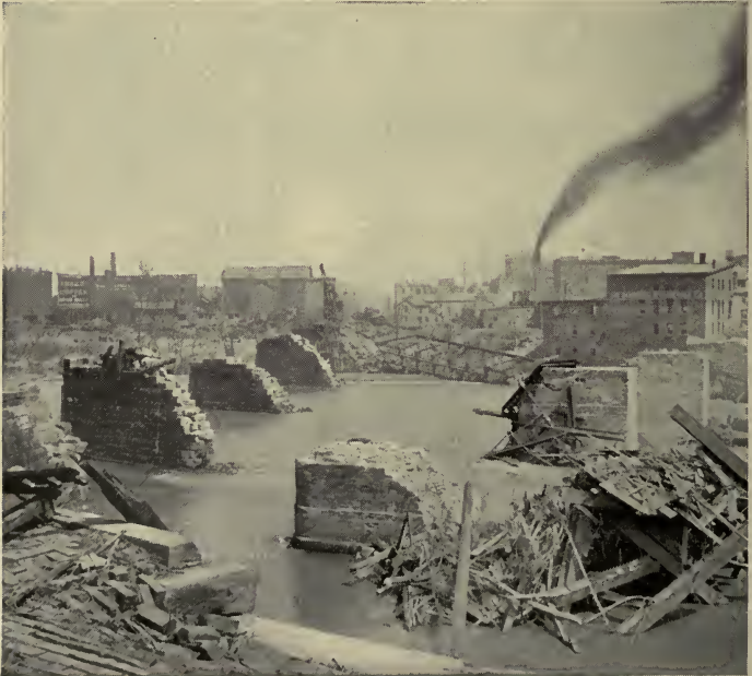
Zanesville, Ohio. Pennsylvania Bridge Over Muskingum River
