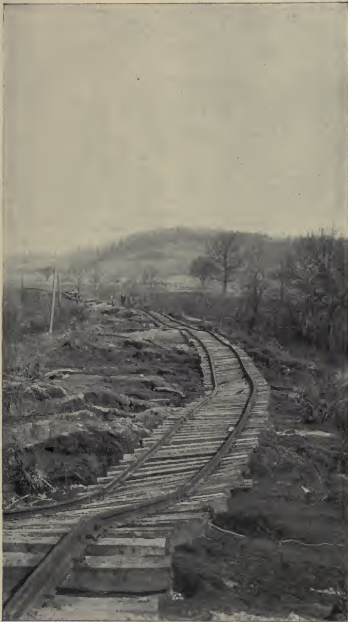
North of Bridge No. 123, North of Warsaw, Ohio. Track was, Before the Flood, on a High Embankment
