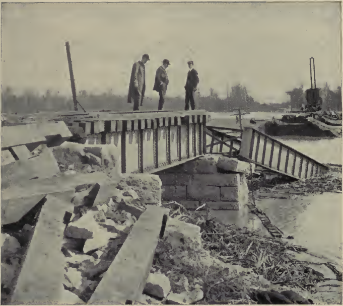
Bridge No. 37, One Mile North of Rockford, Ind.
