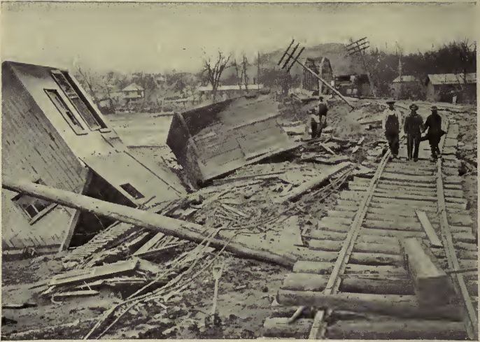
Zanesville Terminal Railroad, Licking Bridge in Background
