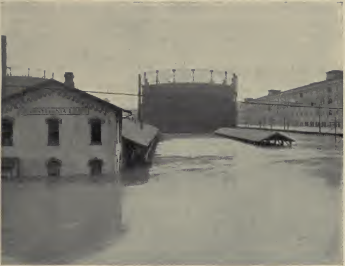
Cincinnati—Smith Street Freight Station when the Ohio River was at its Highest Stage
