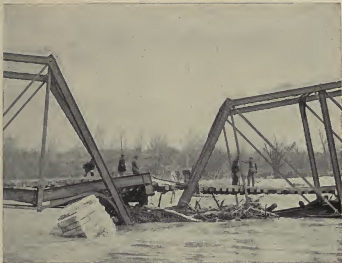
Bridge No. 48, Three-quarters of a Mile East of Somerville, Ohio
