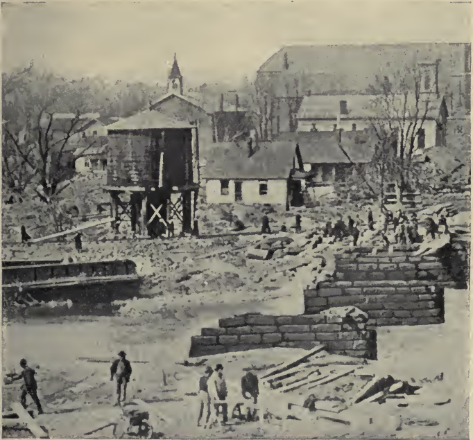
William Street Bridge, Delaware, Ohio
