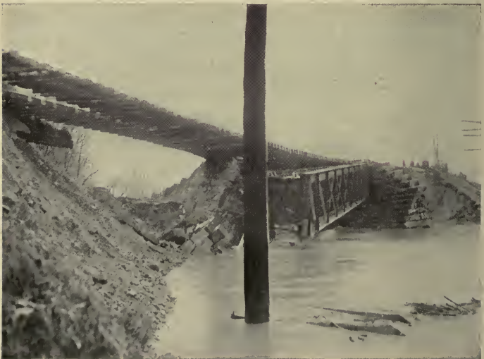
Bridge No. 146, Over Rocky Fork, Eastern Division
