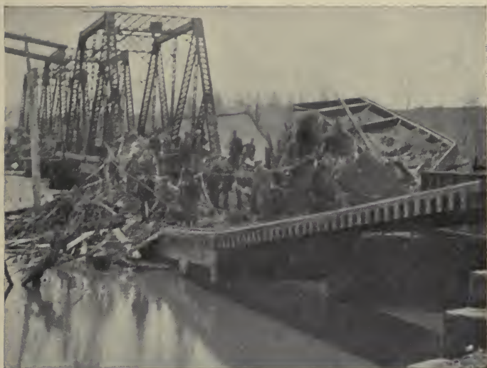
Bridge No. 68, Brink Haven, Ohio
