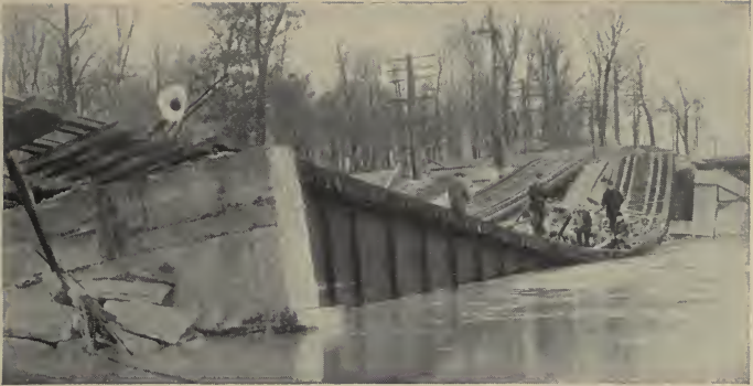
Bridge Over Black Fork, which had to be Entirely Replaced
