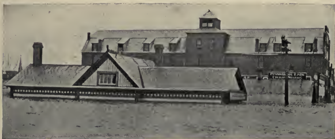
Marietta (Ohio) Passenger Station. Water had Receded One Foot
