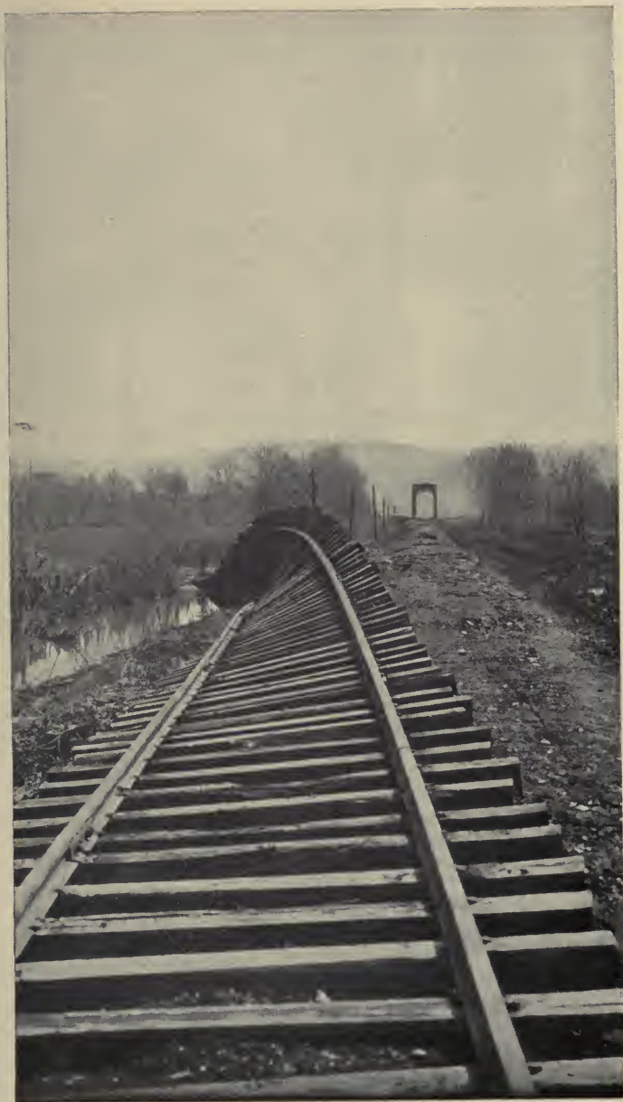
Bridge No. 120, Over Killbuck Creek, Akron Division
