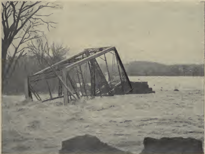
Bridge No. 83, Over Kokosing River. Steel Work of Both Spans Gone Out. One Pier and One Abutment Destroyed
