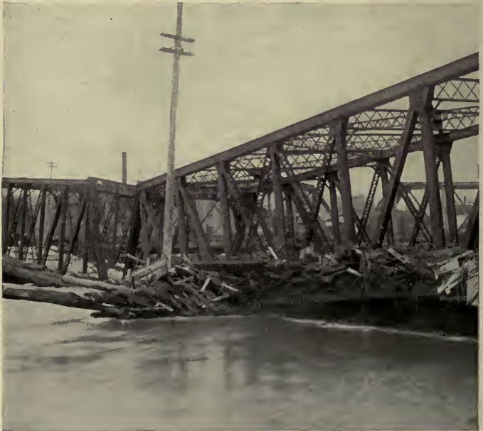
Street Bridge, Sharon, Pa.
