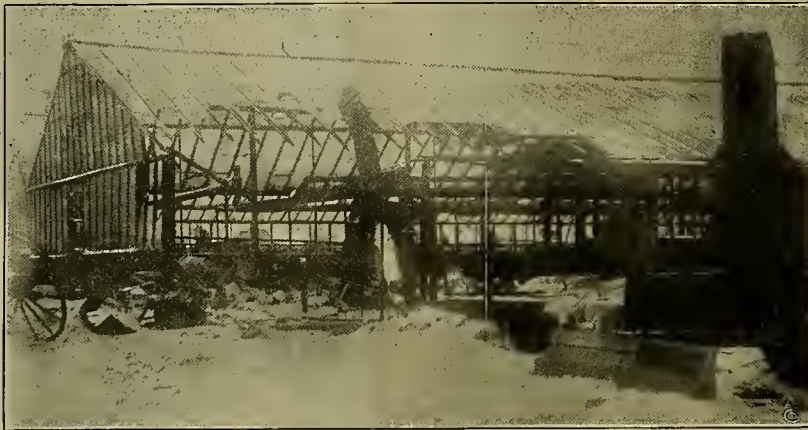
AFTER THE FIRE AT DANVILLE FLORAL CO., DANVILLE, ILL., JANUARY 7, 1912.
