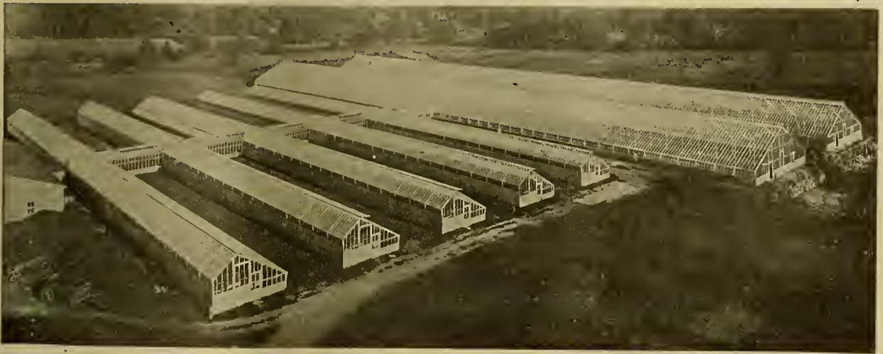
Rowayton Greenhouses at Rowayton, Conn.
