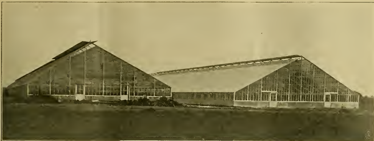
THE JOS. HEACOCK CO.'S PLANT AT ROELEFS, PA.
