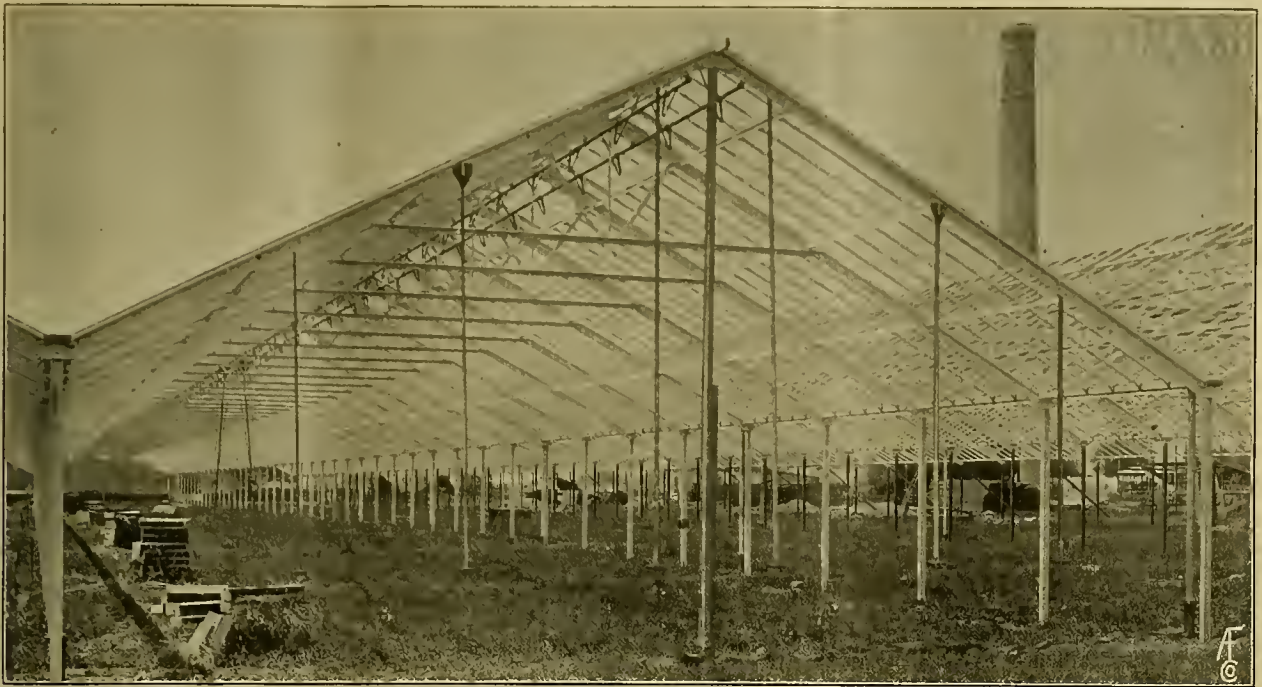
E. G. HILL CO.'S NEW RANGE AT RICHMOND, IND. Interior View of One of the Houses in Course of Construction.
