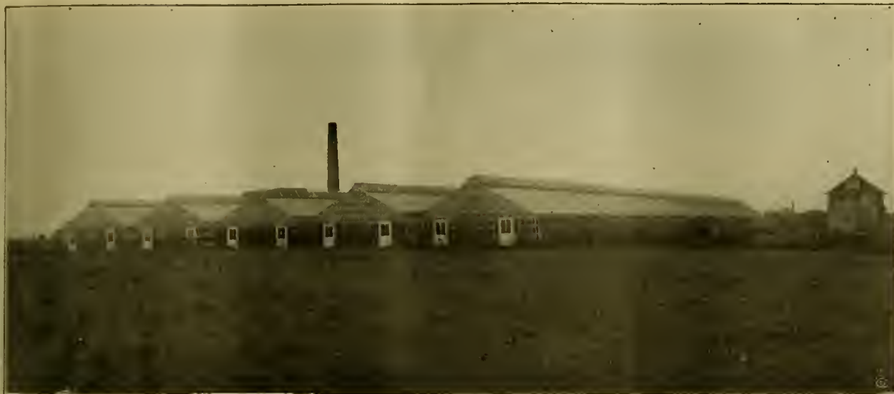
EXTERIOR VIEW OF F. STIELOW'S RANGE AT NILES CENTER, ILL.
