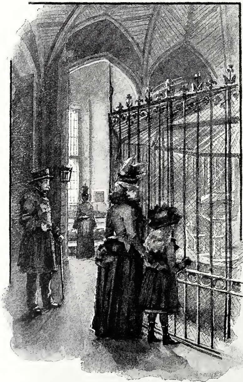
Interior of the Wakefield Tower.
