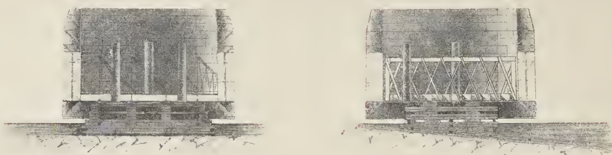
CAISSON ON LAUNCHING SLIPS
