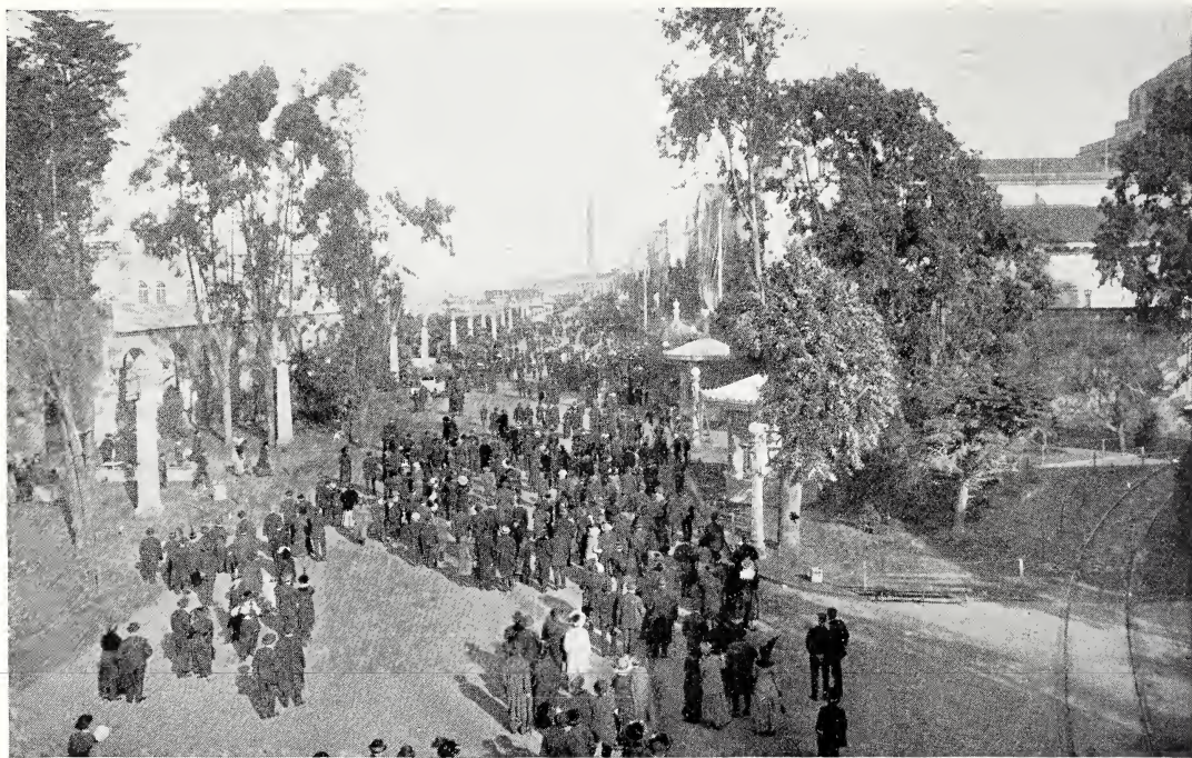
THE ESPLANADE FROM ADMINISTRATION AVENUE
