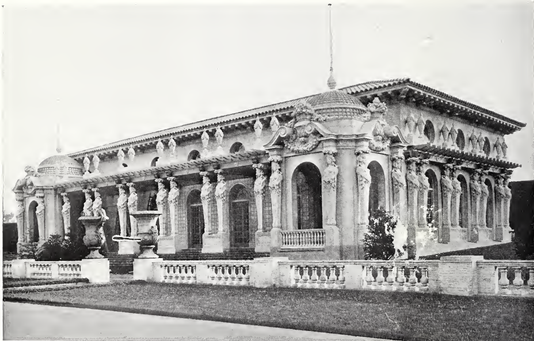
THE PRESS BUILDING
