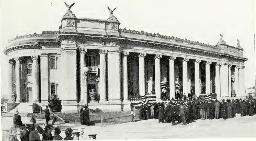
THE WASHINGTON STATE BUILDING
