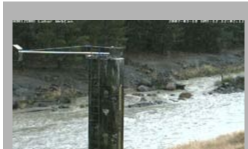
Before the lahar at midday (UTC+12) at the Tangiwai Bridge at Whangaehu Valley.
