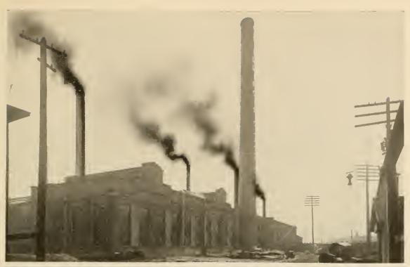
New Power House of the Illinois Glass Co., Alton, Illinois. The Large Stack Carries the Gases From Four 300-Horse-Power Boilers.
