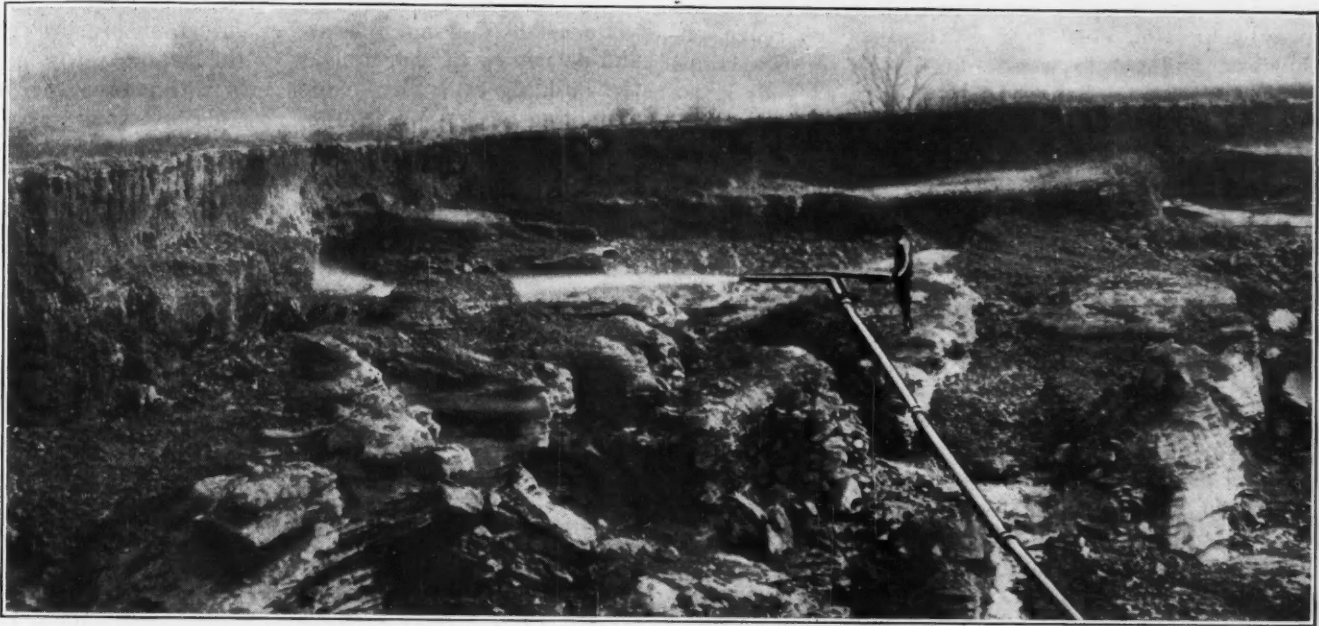
HYDRAULIC MINING AT PROPERTY OF BLUE GRASS PHOSPHATE CO., SOUTH OF MOUNT PLEASANT, TENN.
