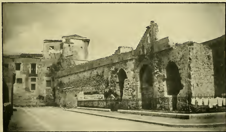
INSIDE THE MONTALTO BASTION.
