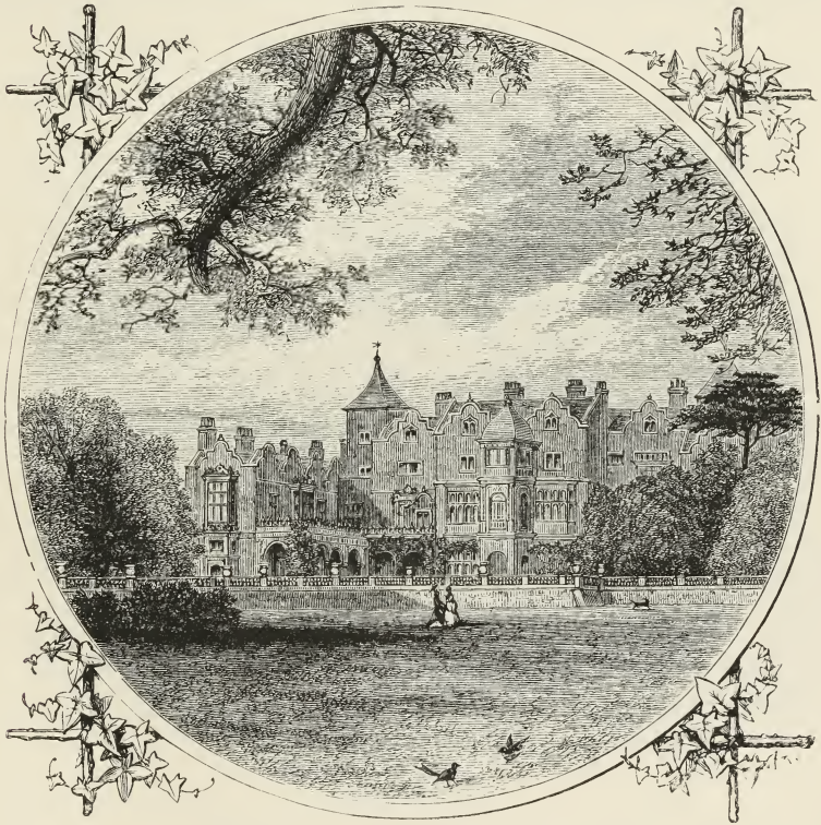
South view of House, from Drive.
