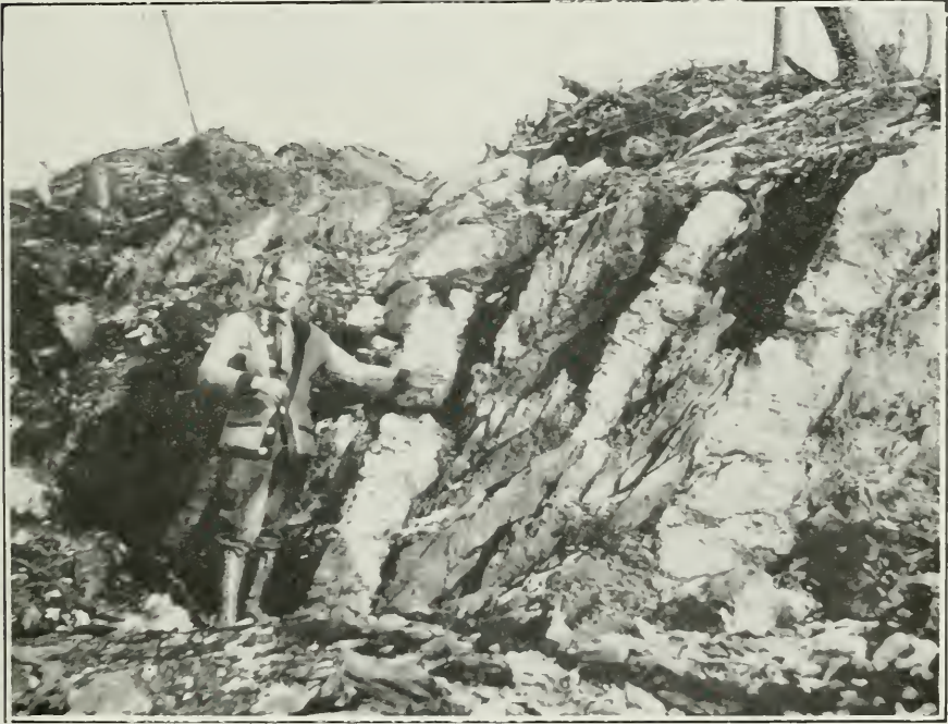
Narrow quartz veins in Keewatin carbonate schist at Dome property. Nov. 1910.
