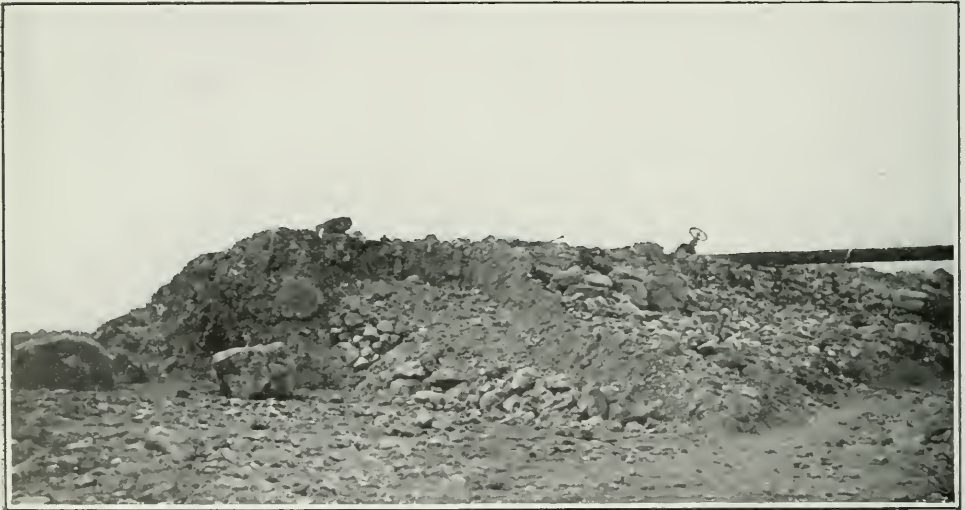
Cross section of earthen dam between upper and central parts of unwatered area, showing the main conduit conveying air from compressor plant.
