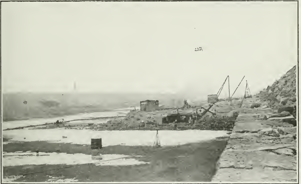
Stony island "Dry Cut"—a general view taken from the north showing one of the three steam shovels at work with dump skip lowered alongside
