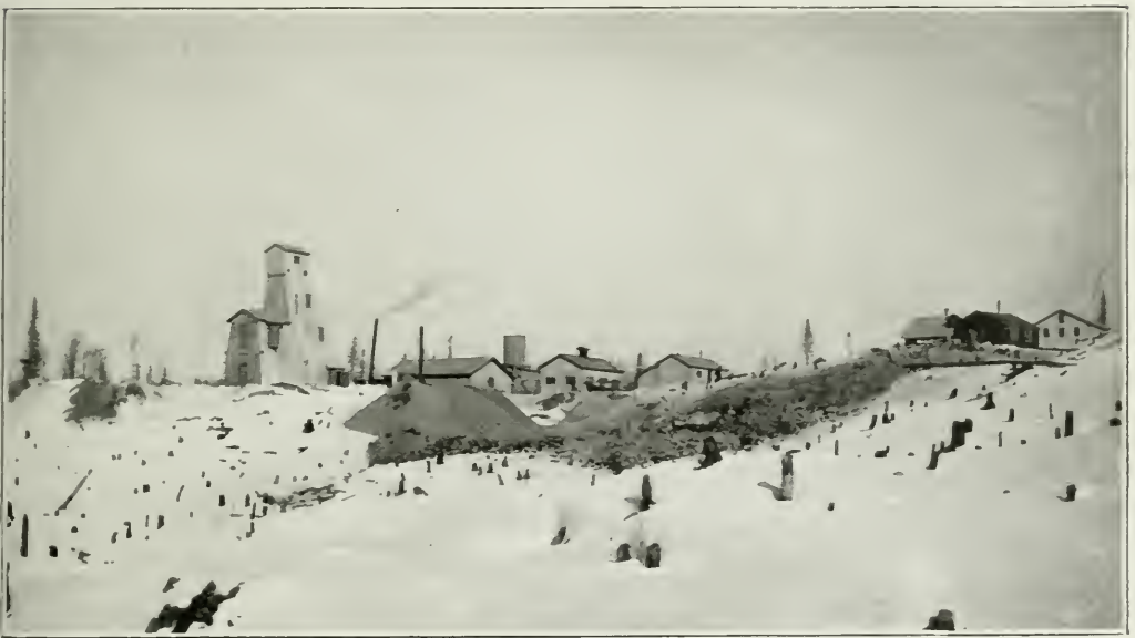
Vipond mine. March, 1912. Preparing site for mill.
