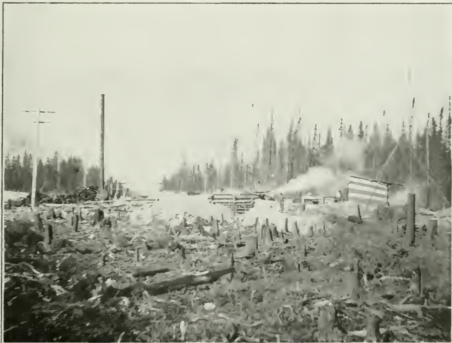
North Dome mine, showing power transmission line; shot drill in operation. Oct. 1911.
