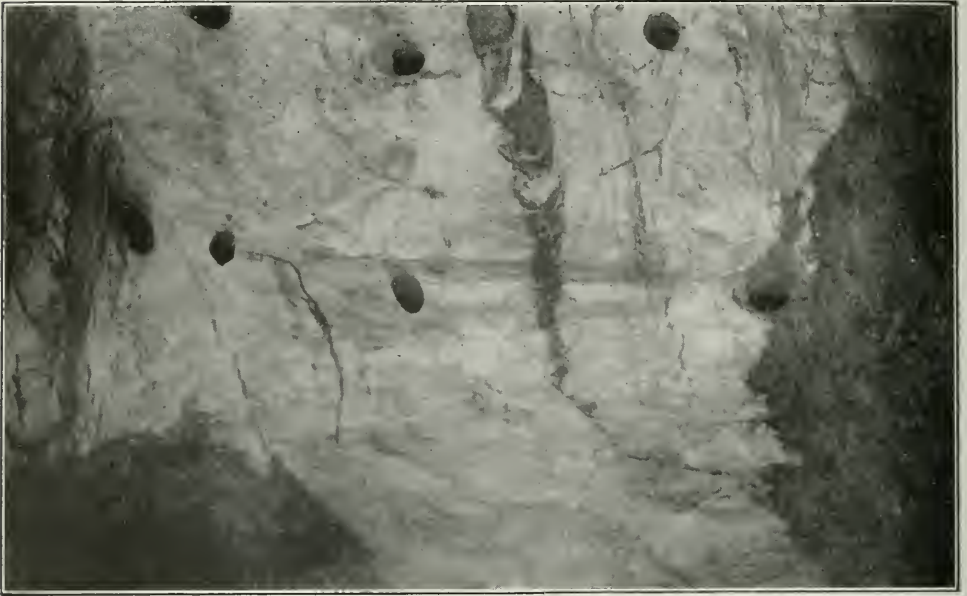
Quartz vein on 100-foot level, McEnaney mine. The dark spots are drill holes.
