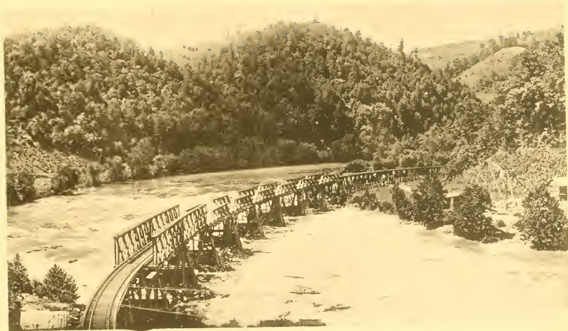
SOUTHERN RAILWAY BRIDGE OVER THE FIBERO DRAIN BY STARBUCK.
