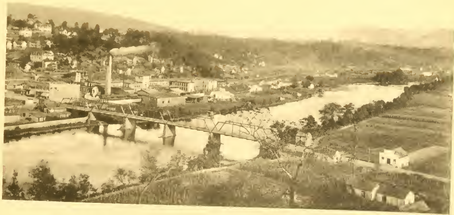
UNION BRIDGE ACROSS THE FRESH BRANCH
