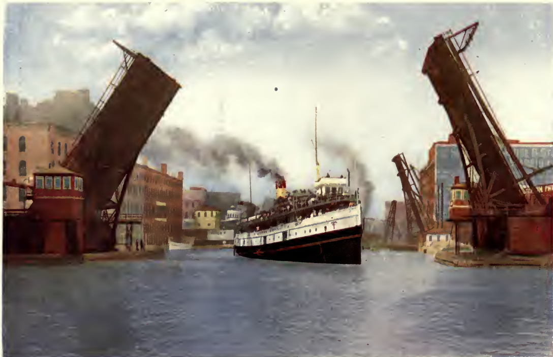
STATE STREET BASCULE BRIDGE LIFTED FOR STEAMSHIP SOO CITY.
