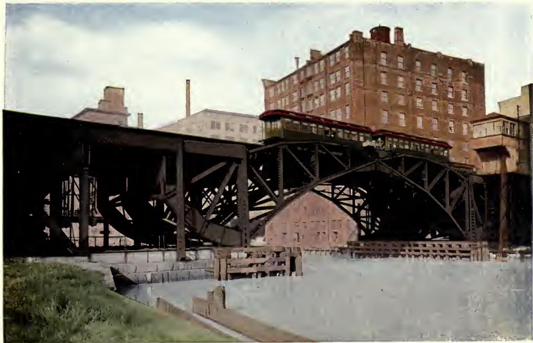
METROPOLITAN TRAINS CROSSING BASCULE BRIDGE OVER CHICAGO RIVER.
