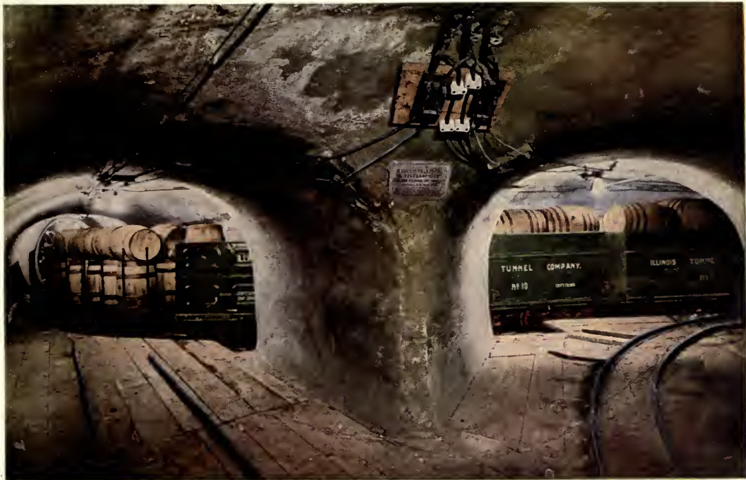
UNDERGROUND TUNNEL AT STREET INTERSECTION, SHOWING LOADED FREIGHT CARS.
