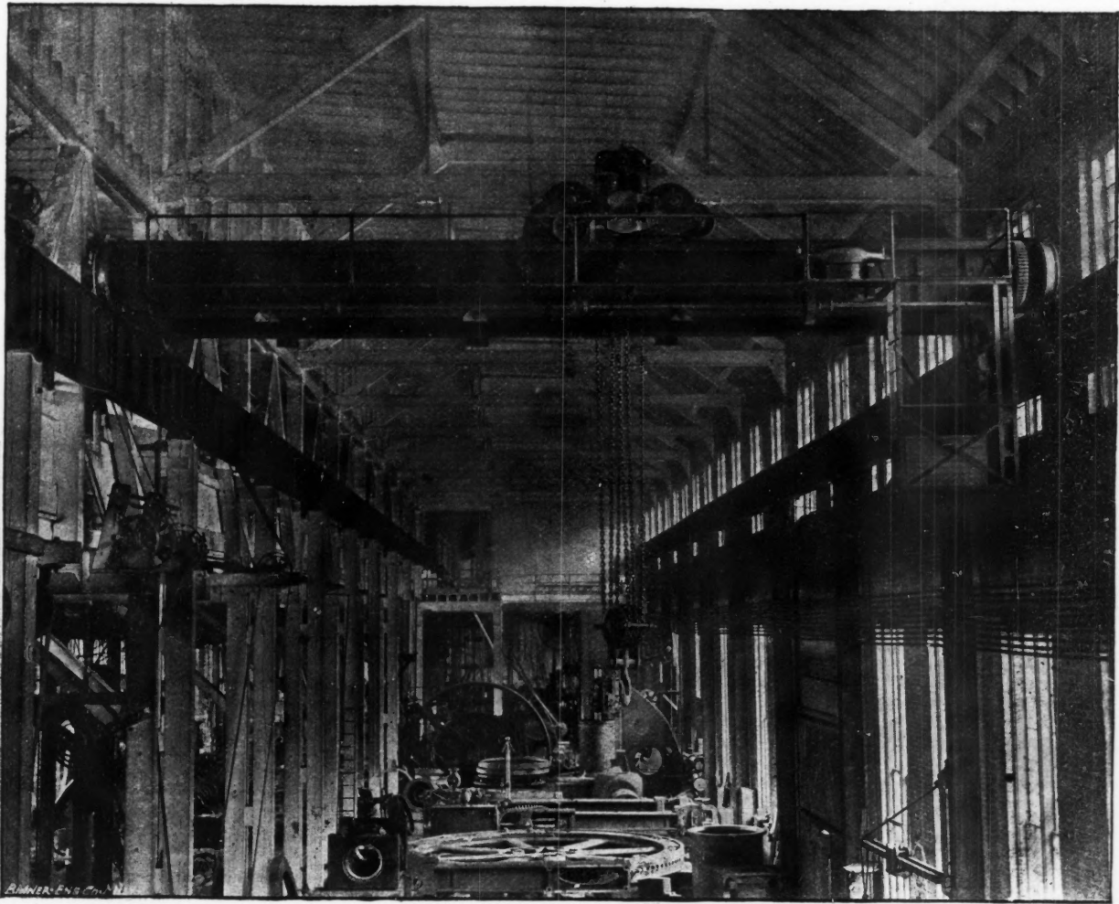
SHAW ELECTRIC TRAVELING CRANE IN THE WORKS OF THE E. P. ALLIS Co., MILWAUKEE, WIS.
