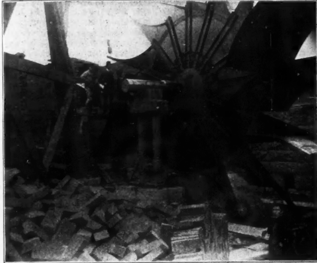
FAN IN COURSE OF ERECTION.
