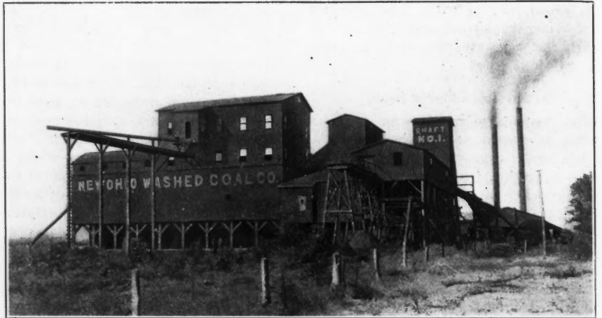
LUHRIG WASHERY OF THE NEW OHIO WASHED COAL COMPANY AT CARTERVILLE, ILLINOIS. CAPACITY 60 TONS PER HOUR
