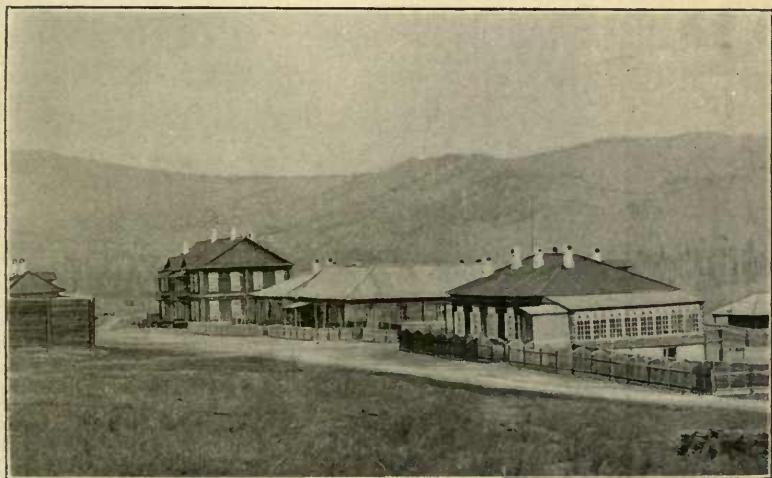
GOVERNOR'S HOUSE, BARRACKS, AND PART OF OLD PRISON, AKATUI. The only place in Siberia where political convicts are now sent to hard labour in the mines.
