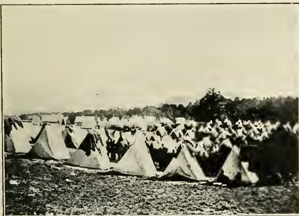
THE CITY OF TENTS. The Army of the Potomac encamped in readiness for the forward movement on Richmond. These comfortable canvas houses were transported by the army wagons. The Confederates had no such complete shelter during the spring of 1862, which was remarkable for the inclemency of the weather.
