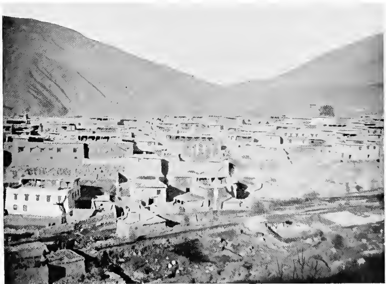
BATANG, LOOKING NORTH
