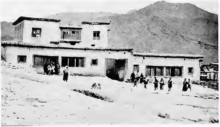
OFFICIAL'S HOUSE AT DRAYA JYAMDUN
