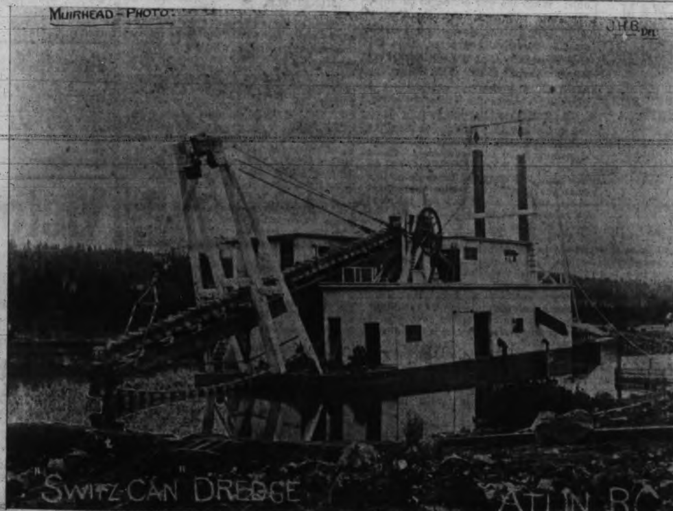
MODERN DREDGE ON ATLIN CREEK.
