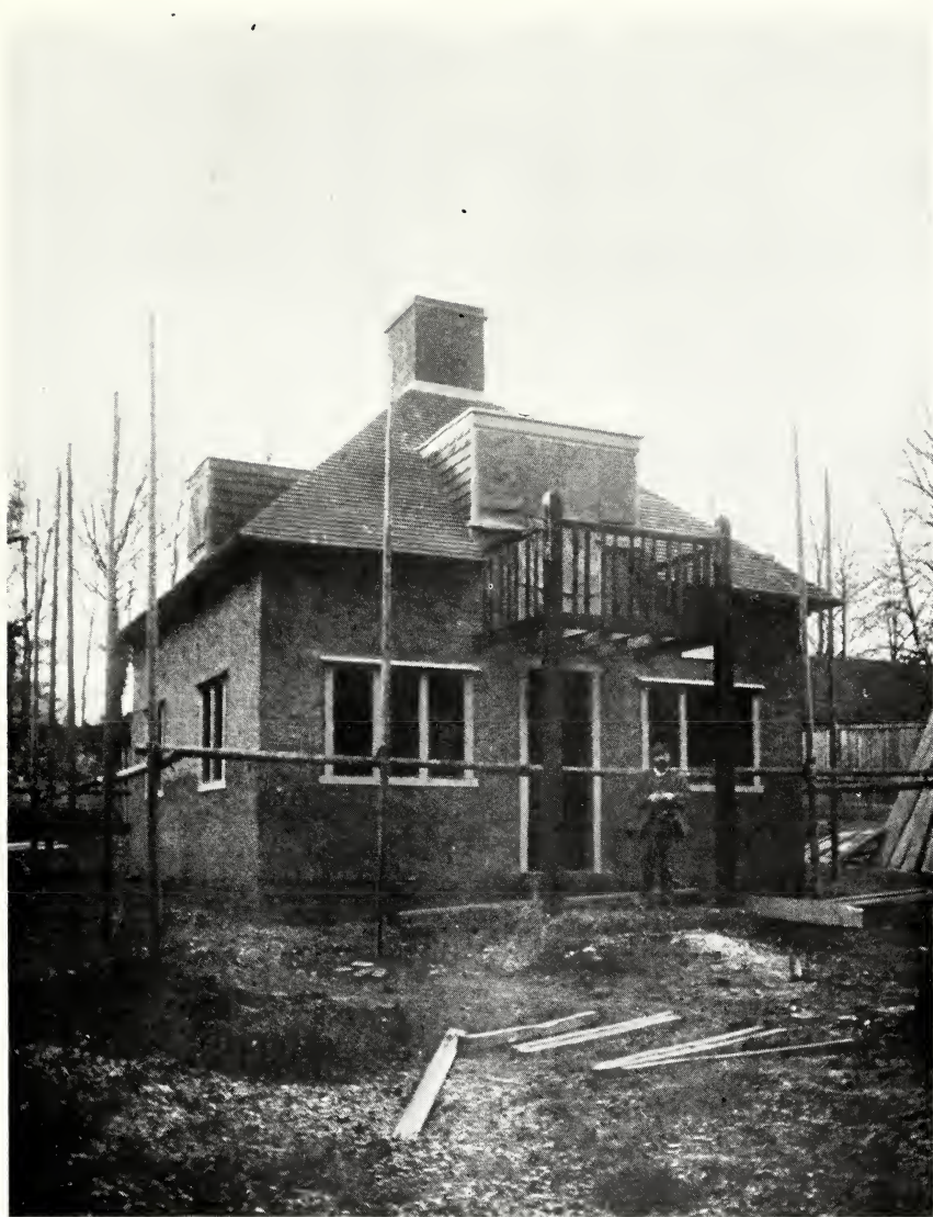
Appendix No. 10. The Nursing Cottage at Findon (in construction).
