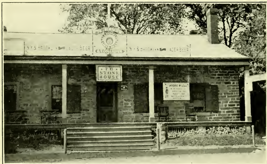
André Prison House, After Restoration.
