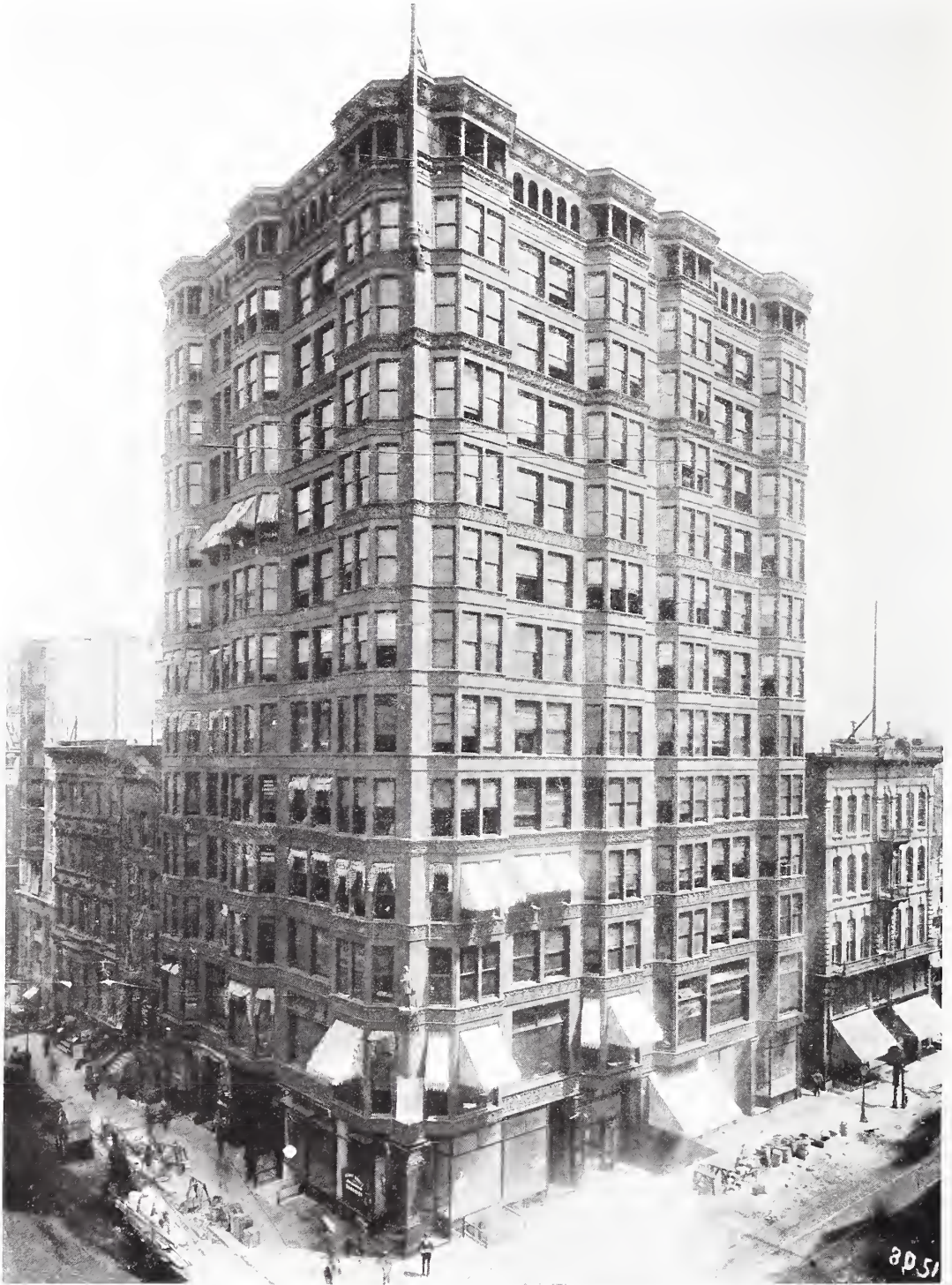
The Tacoma Building. A Milestone in American architecture. The first building in the world of skeleton steel construction Holabird and Roche, Architects.
