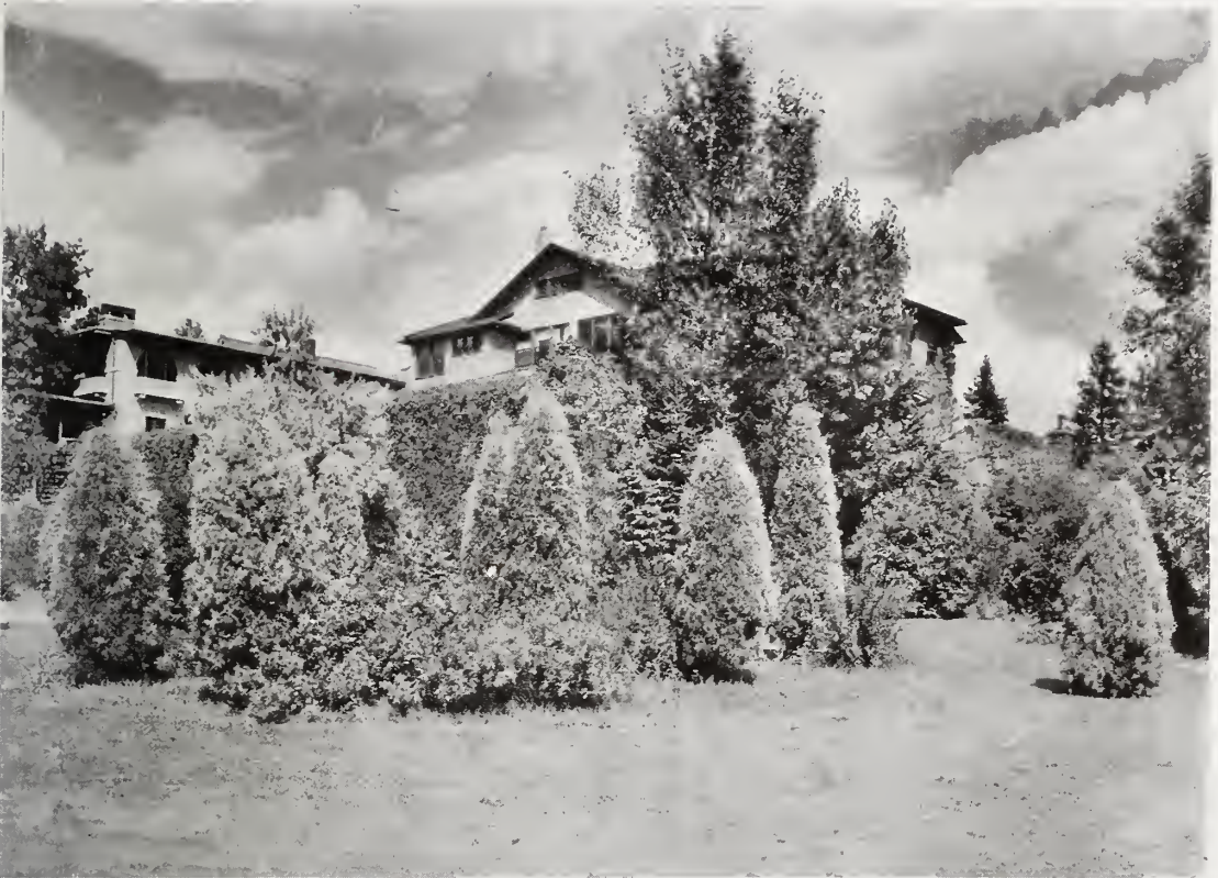
Photograph of H. L. Standley, Colorado Springs
