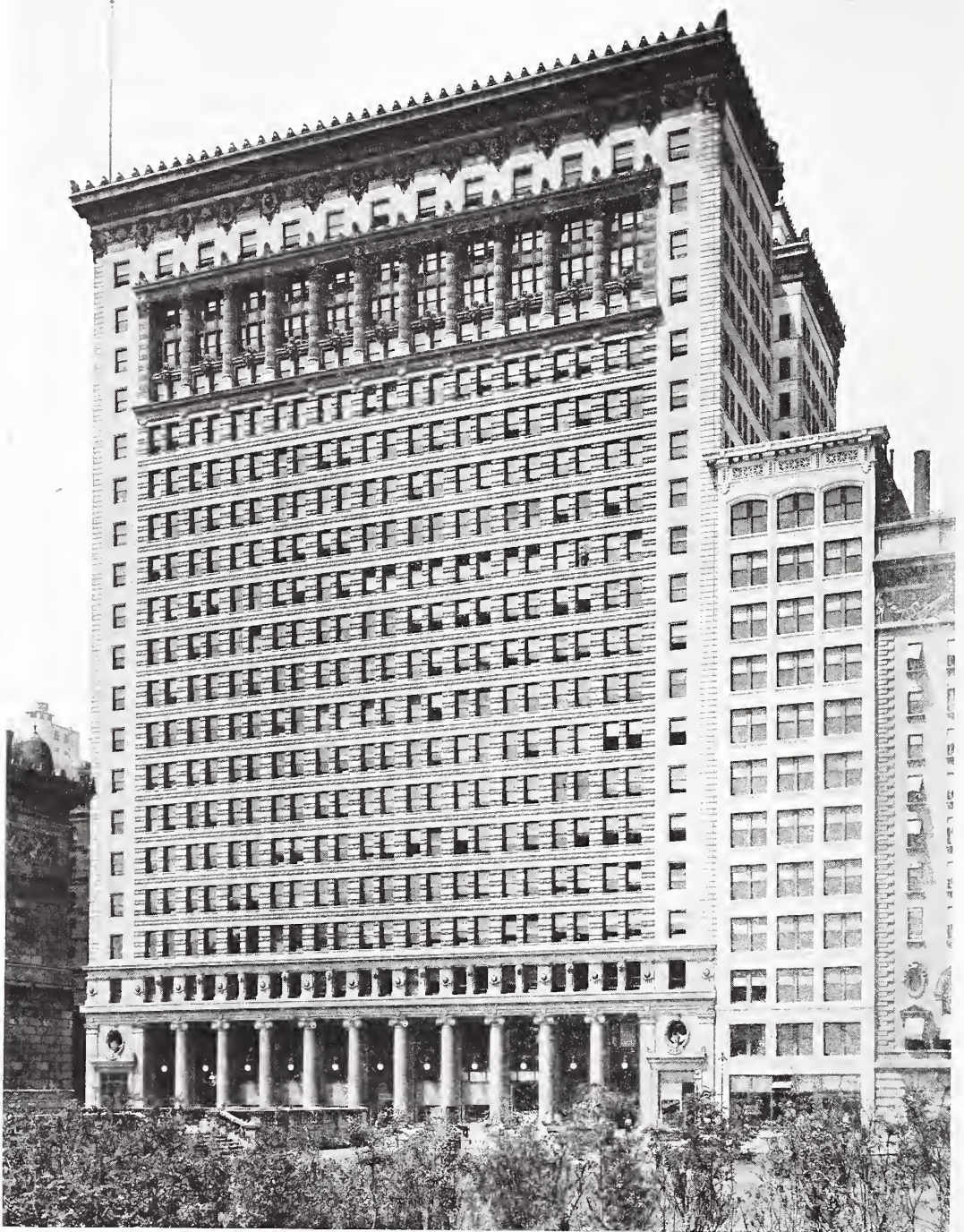
The Peoples Gas Building—a brilliant example of modern eclecticism. The Roman detail forms an interesting texture. The first story granite columns are a solecism—they support nothing but themselves. Graham-Anderson, Probst and White, Architects.
