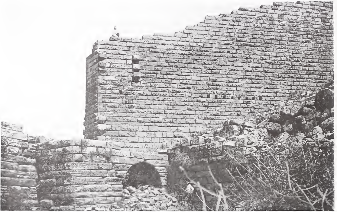
Western Transverse Wall, showing a high grade of stone-work, and a Gateway with a corbelled arch.
