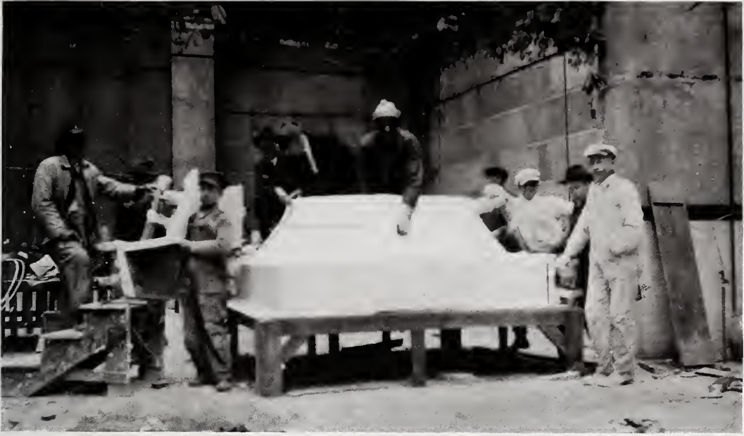
OPENING THE MOULD OF THE CAPITALS.
