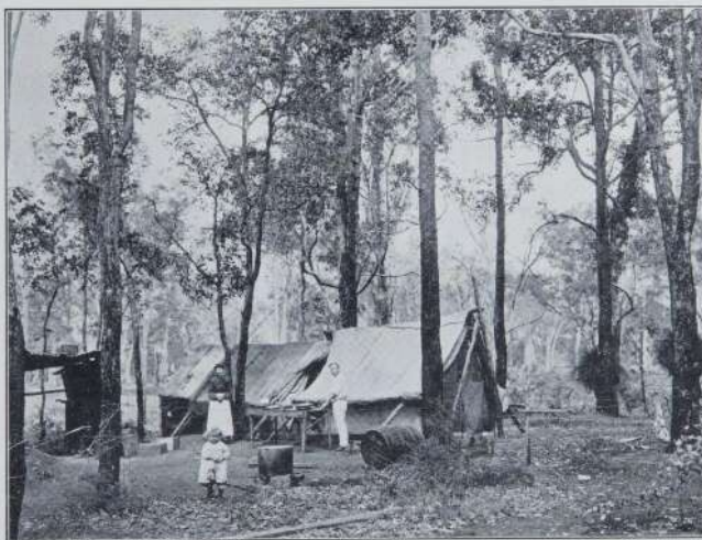
NEW SELECTOR AT BRUNSWICK (SOUTH-WEST).
