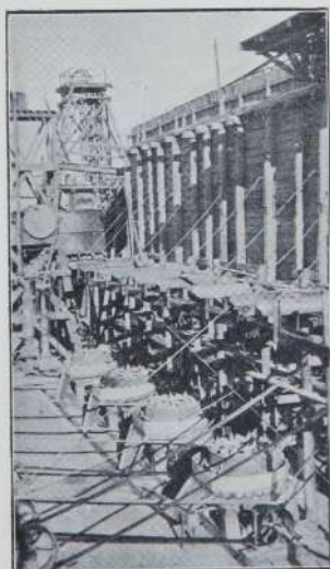
HUNTINGDON MILLS, ORE BINS, AND POPPET OVER MAIN SHAFT.
