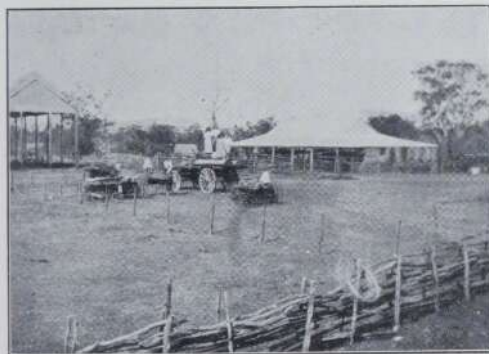
OUTBUILDINGS AT "NOOMBLING."
