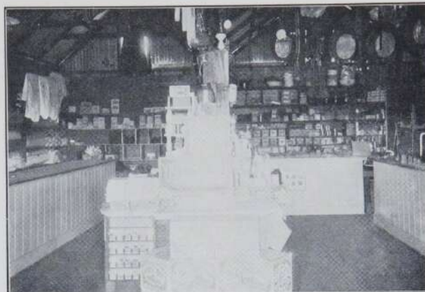
Photo by W. E. Elston. INTERIOR OF STORE.
