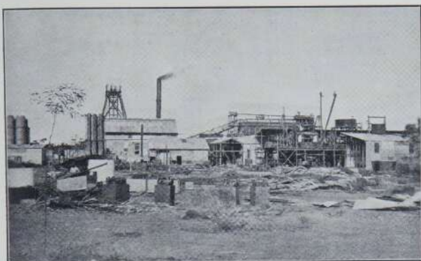
VIEW OF SURFACE PLANT, VICTORIOUS MINE, ORA BANDA.
