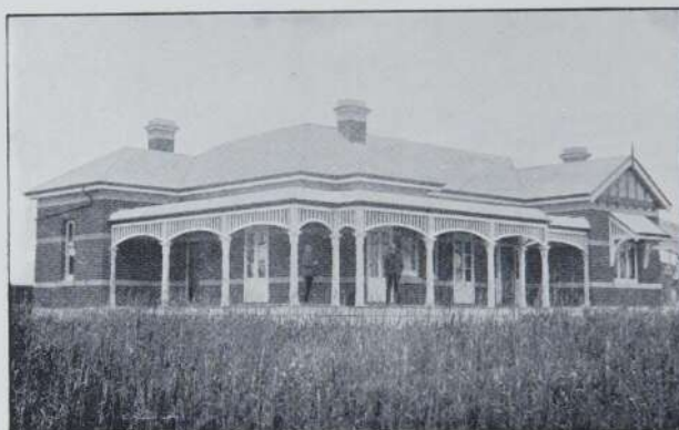
"TELYARUP," RESIDENCE OF MR. M. CORBETT, BROOME HILL.
