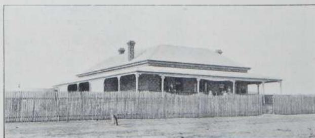
MR. T. REYNOLDS' RESIDENCE, MECKERING.
