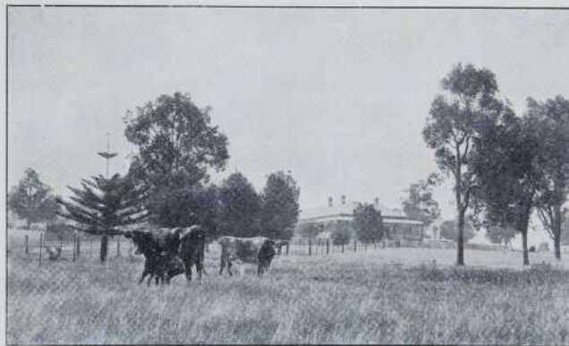
Photo by Greenham & Evans. "STRATHALBYN" HOMESTEAD.
