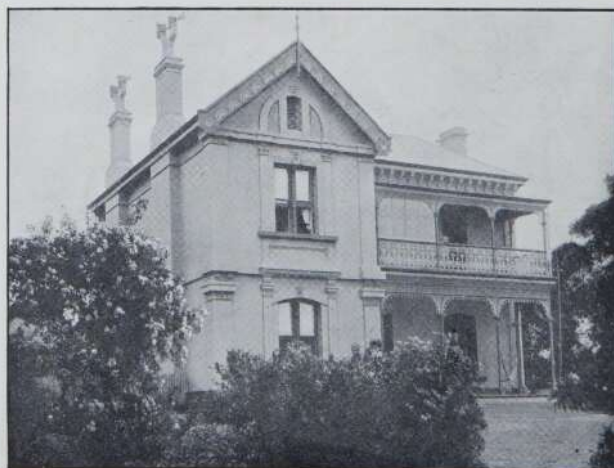
"HILLSIDE," MR. A. Y. HASSELL'S RESIDENCE, ALBANY.
