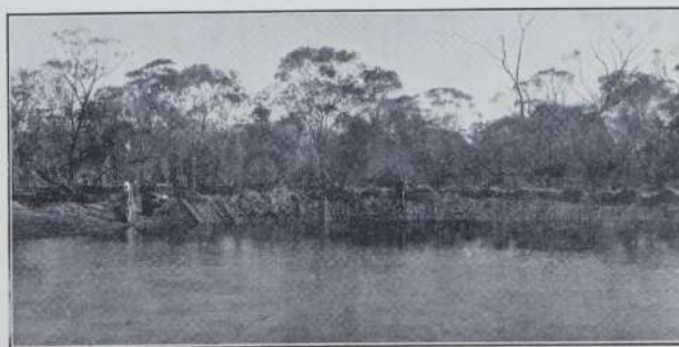
DAM (750,000 GALLONS CAPACITY) ON THE WARREN ROAD.
