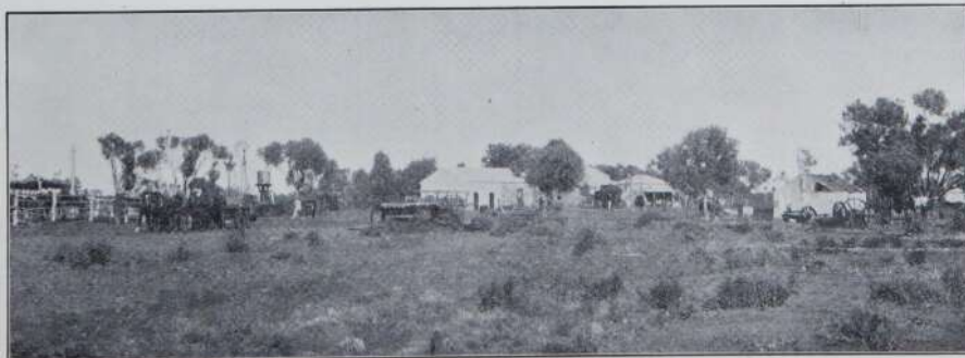
OLD HOMESTEAD AT "YANREYREDDY" STATION (PARTLY DEMOLISHED).
