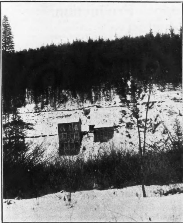
INTERNATIONAL MINE, NEAR ORO GRANDE, CENTRAL IDAHO
