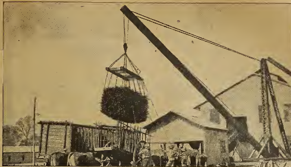
The cane is then unloaded, and dumped on a long feeder, which starts it on its journey through the mill
