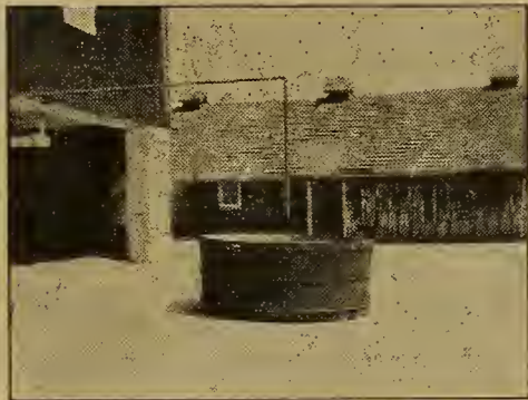
A barnyard paved with concrete keeps the cows cleaner and enables the regular work to go on even in wet weather
