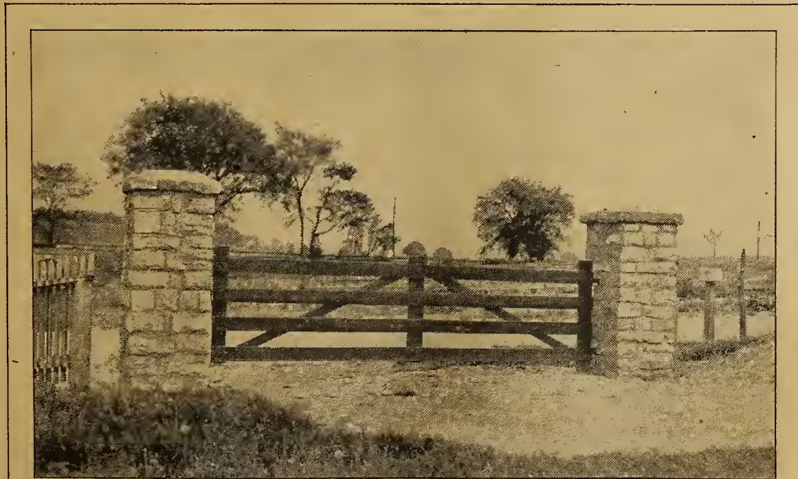
What you see here is only a beginning. An ornamental metal gate will replace this wooden one, and an evergreen hedge will line the lane on both sides
