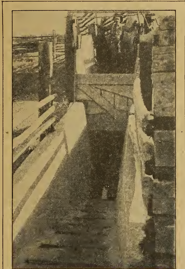
Looking down on a farm-size concrete dipping vat. The gate slides up to admit the stock
