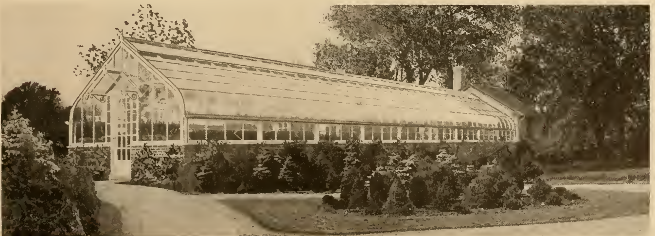
After seeing the Mackenzie house at Narragansett Pier, we took a Saturday afternoon off, and ran over to the Philadelphia suburbs, to see this three compartment house, seventy-five feet long.
