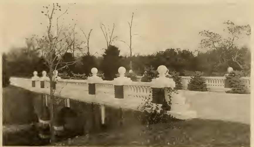
Bridge on the Bourne Estate, Oakdale, N. Y.
