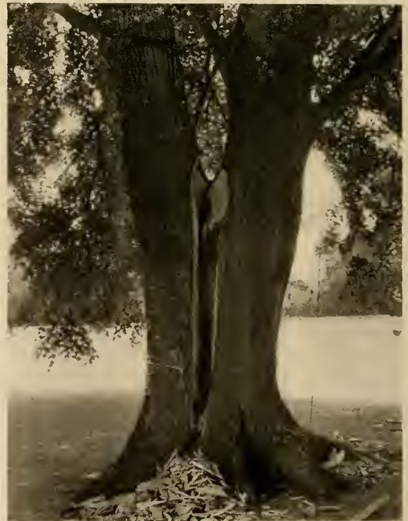
Showing the Decayed Condition of the Tree, After the Surgeons Cut Into Its Trunk.
