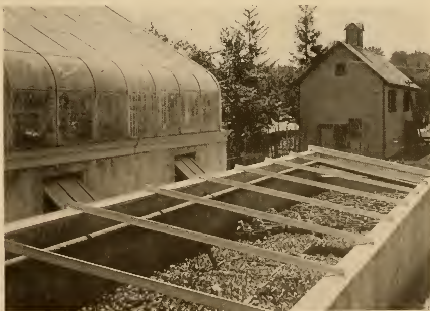
This comes pretty close to being an ideal arrangement of frames, in connection with a greenhouse. You will notice that there is a heating pipe running around the sides. The masonry work is of concrete, capped by cast iron sills, upon which angle iron rafters are bolted. It will last as long as the greenhouse. Note how it is filled with potted plants and bedding ones in flats, ready for transplanting in the outdoors garden.
