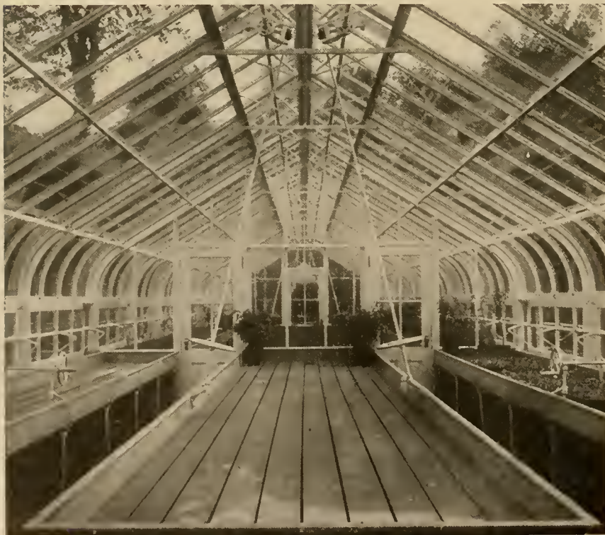
This is the interior of the two compartment house that we showed to Mr. Brown, so that he could see the construction arrangement of the benches.
