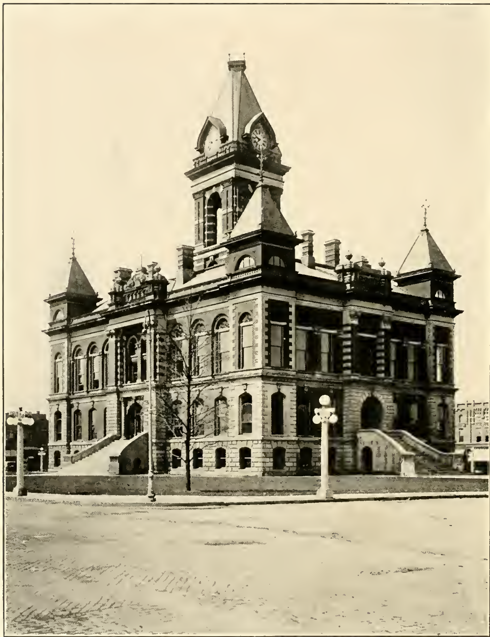
GIBSON COUNTY COURT HOUSE.
