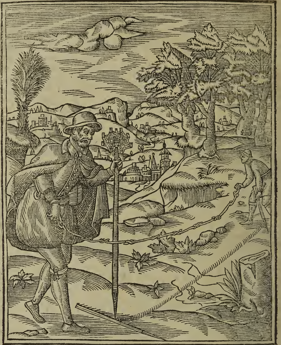
How to reduce all sorts of grounds into a square for the better measuring of it.
