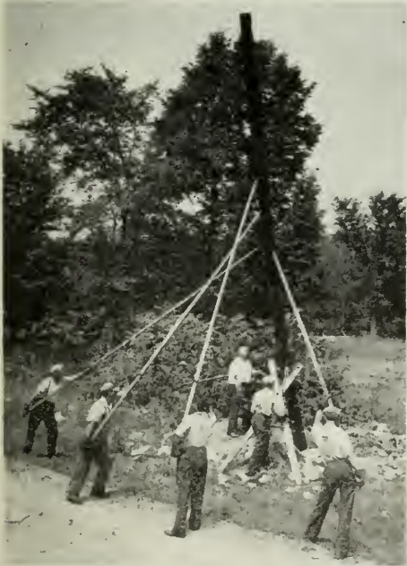
Surveying the Route Erecting the Pole
