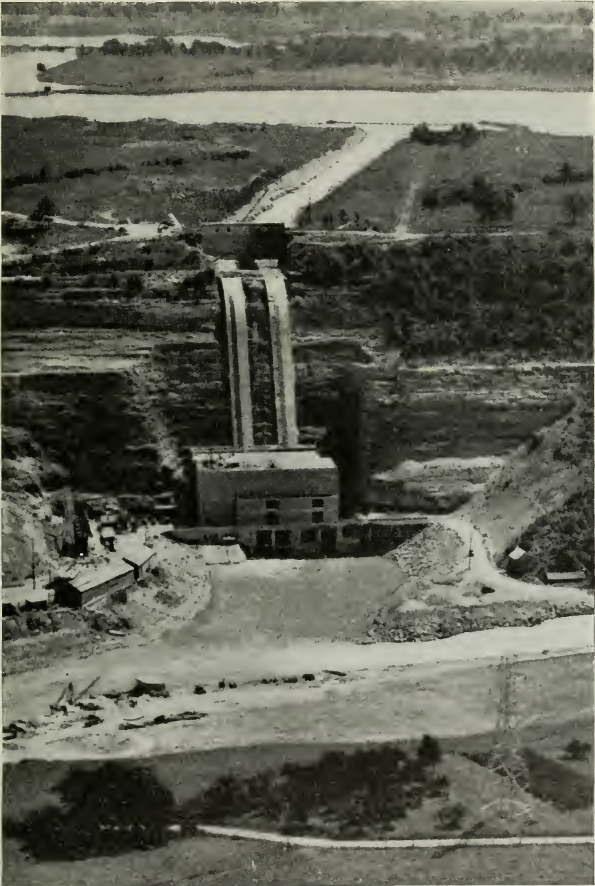
DeCew Falls 150,000-horsepower station on Twelve Mile creek, near St. Catharines. The second unit, 77,000 horsepower, went in operation in September, 1947
