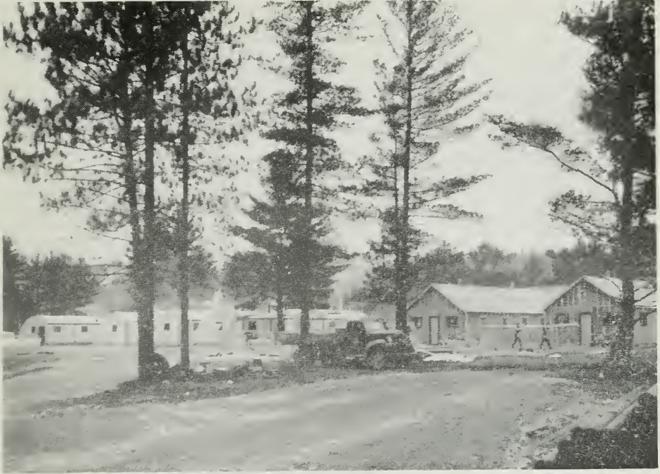
TUNNEL Construction camp late in 1947 at this 56,500-horsepower project on the Mississagi river. Also see frontispiece
