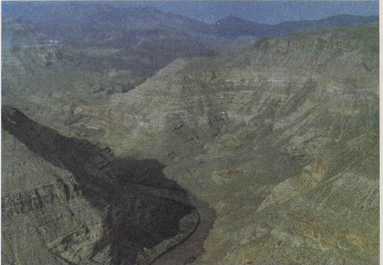
Aerial view of the Virgin River Gorge in Starvation Point WSA (005). This WSA is recommended for wilderness designation by the Enhanced Wilderness alternative.
