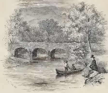
GARAMEEN BRIDGE, KILLARNEY.
