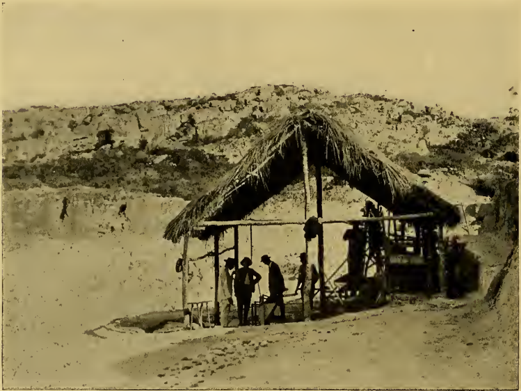
FIG. 21.—The pit of Serrinho. A shallow depression in the Caraça quartzite which was partially filled with diamond-bearing conglomerate. The conglomerate and beautifully white kaolin are seen in the bottom of the excavation. The final washing operations to recover the diamonds are conducted in the batêa , or jig, under the thatched roof.
