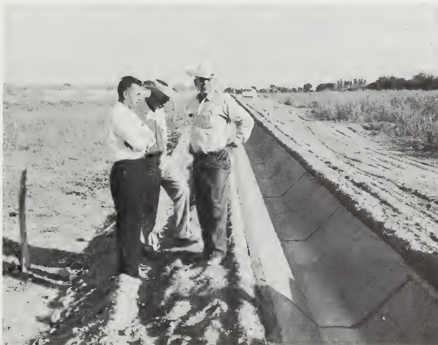
Soil and Water Conservation District supervisors observing recently installed concrete lined irrigation ditch. This practice prevents erosion, saves water, reduces sediment in streams and reservoirs, and facilitates good irrigation system.
