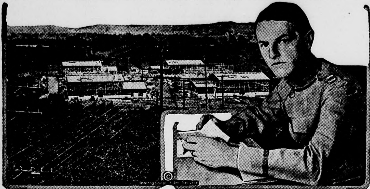
View of the training camp for the national army under construction at Ayer, Mass., and, at right, Capt. Edward Canfield, Jr., U. S. A., who is in charge of the building work there.
