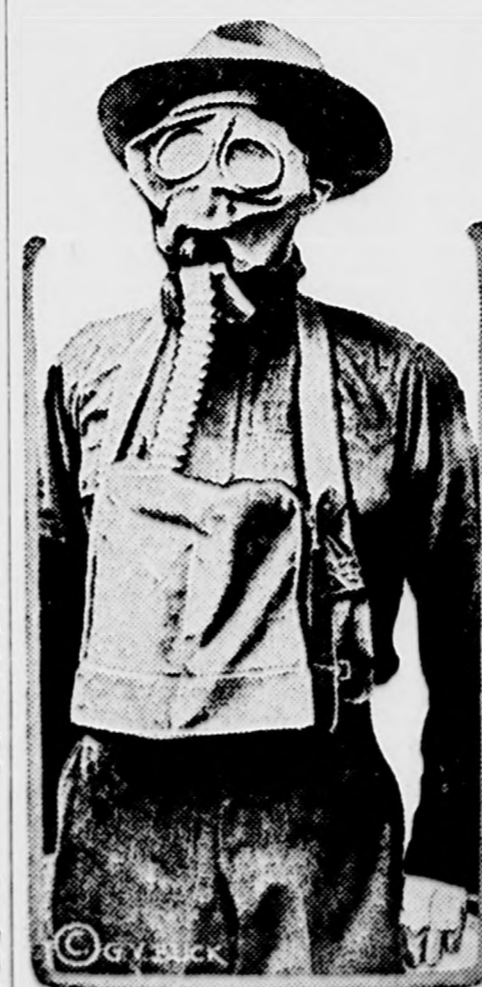
Representative Victor Helatz of Ohio demonstrating a new type of gas mask that may be selected as the mask to be worn by the American troops. The bag must be inflated before use. It is hung over the shoulders and is connected with the face coverings by a peculiarly shaped tubing.
