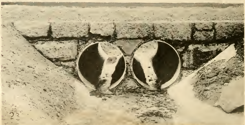
Armco Culverts under the tracks of the Boston & Maine Railway.
