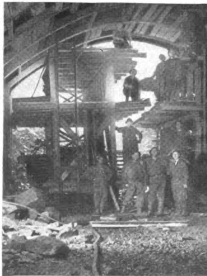
Hard Rock Workers and Jumbos with Drill Platforms
