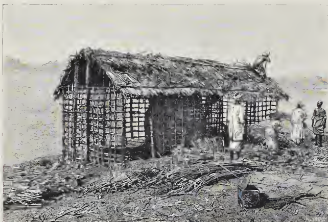
BUNGALOW EN CONSTRUCTION.
