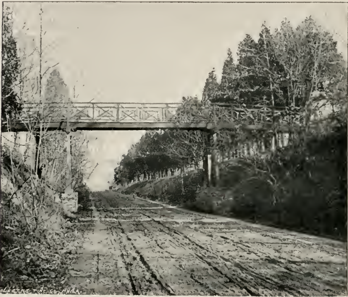
OLD BRIDGE OVER THE RAILROAD.
