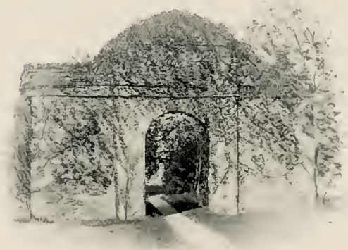
RUINED ARCH OF THE OLD GREENHOUSE.
