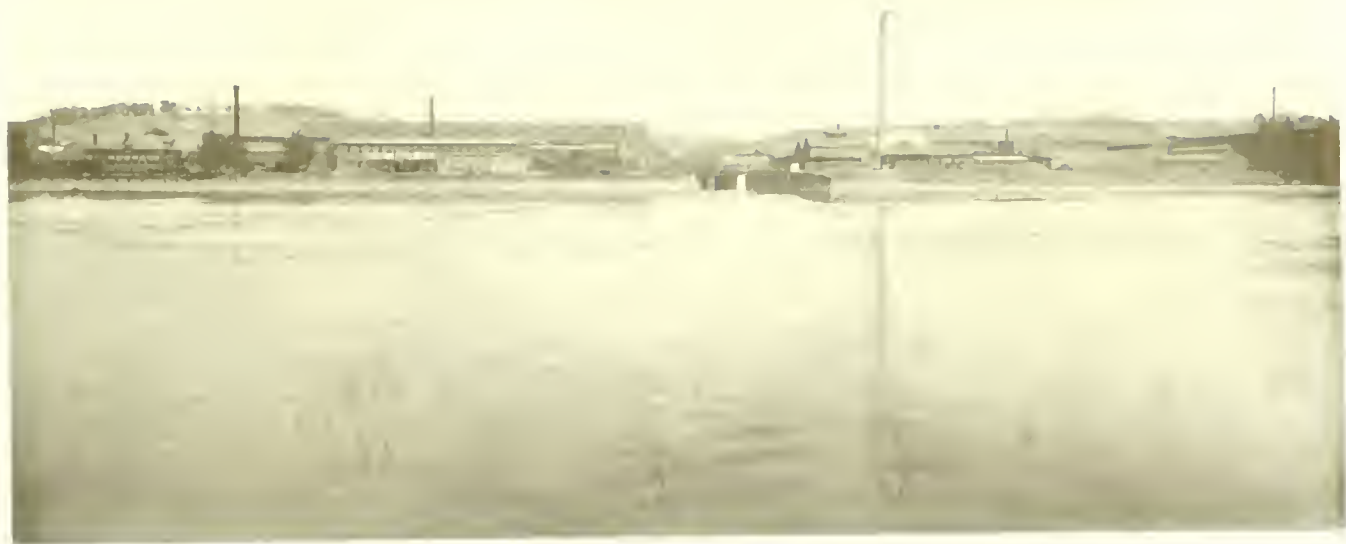
THE HUDSON RIVER In the Lower Part of the City, Showing Some of its Great Iron Industries
