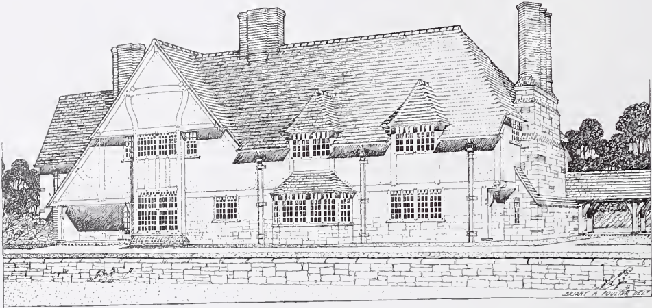
1420. House at Cove, Hants , H. R. AND B. A. POULTER, Architects. Builder: H. W. Yates, Mytchett, Frimley Green, Surrey. (For Plans, see p. 65.)
