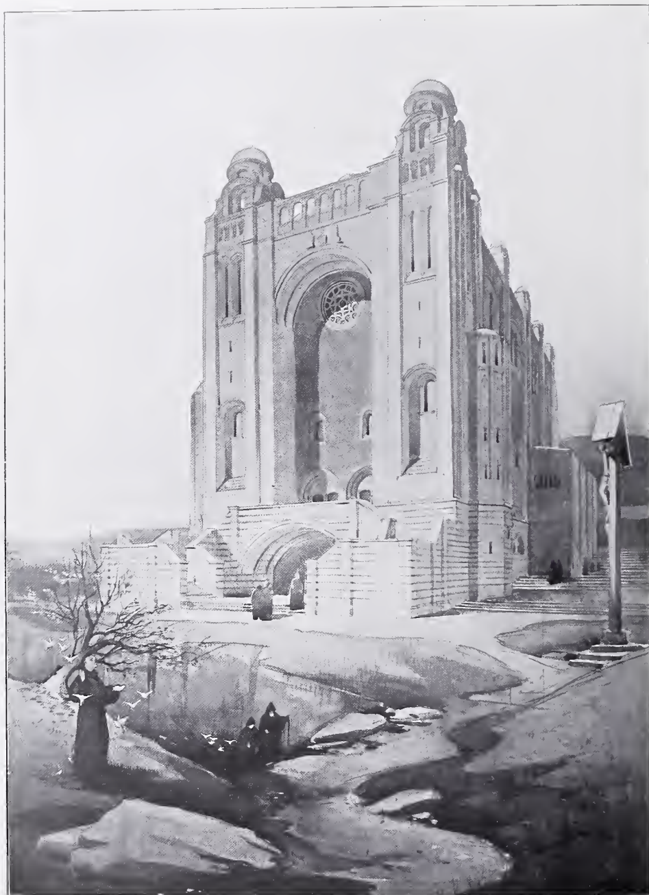
1567. Chapel for the Community of the Resurrection, Mirfield, WALTER TAPPER, Architect.
