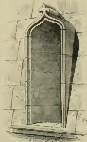
WEEKLEY CHURCH, NORTHAMPTONSHIRE.
