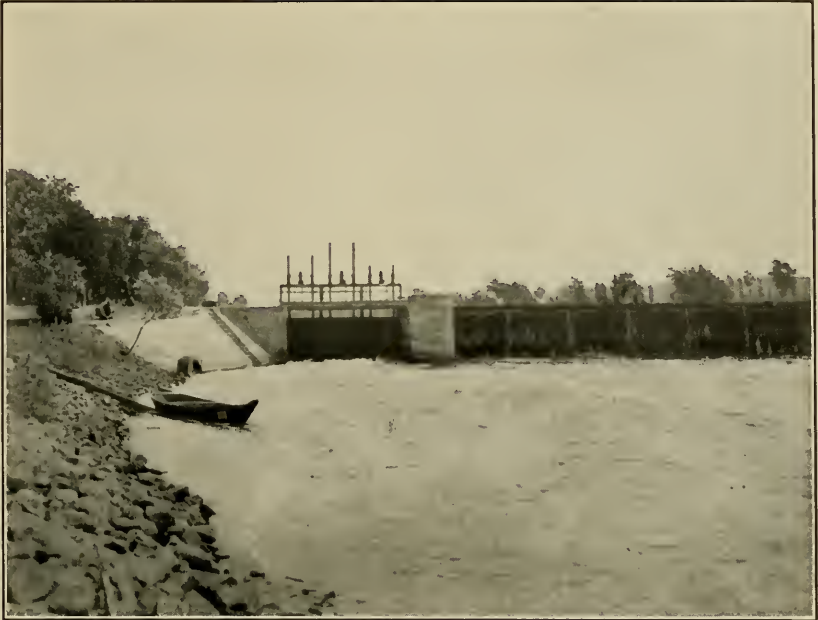
1. The dam in Gruetz on the Havel seen from below; on the right side on the picture the needleweir and on the left side the rampart. Left from it the sloping wall and on its upper edge the trap. (Photographs by Dr. Roehler.)
