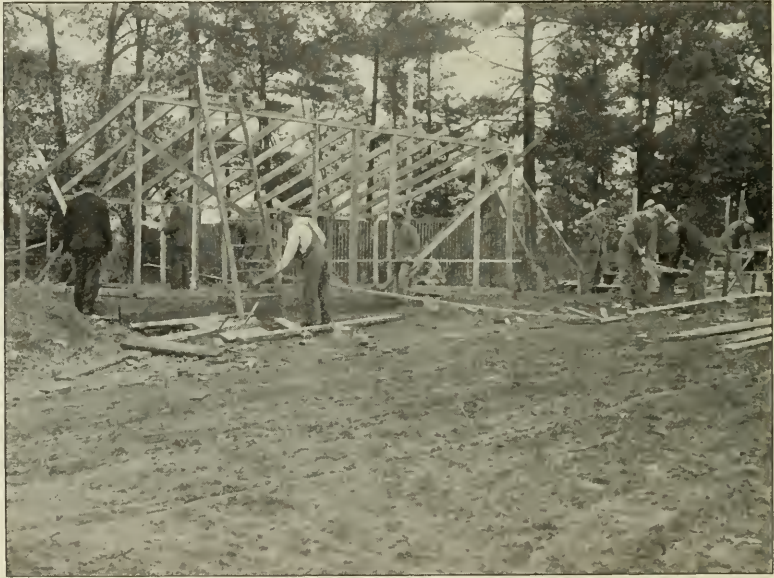
FIG. 347.—Putting up the frame work.
