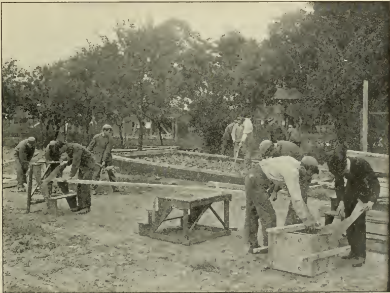
FIG. 346.—Students making the foundation.
