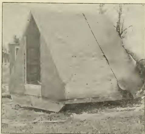
FIG. 72.— Laying the paper roofing.
