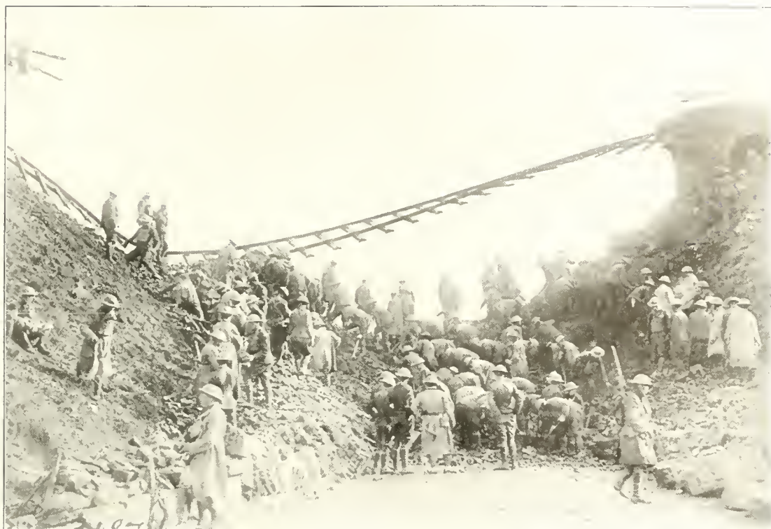
102d ENGINEERS AT ST. SOUPLET BRIDGE
