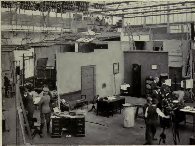
THE CEILING AND FLOOR OF A MODERN EASTERN STUDIO, SHOWING THE LAMPS ON TROLLEYS AND THEIR RELATION TO THE SETS
