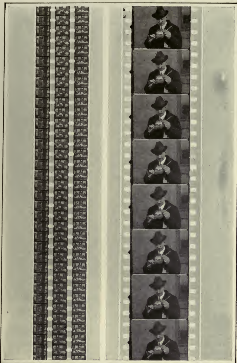
SAMPLE STRIP OF EDISON HOME KINETOSCOPE FILM WITH THREE ROWS OF IMAGES COMPARED WITH STANDARD FILM
