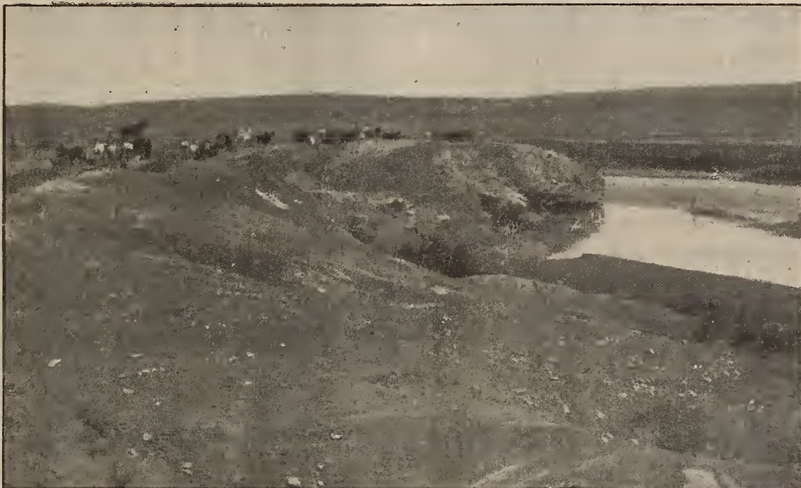
GRADING DOWN THE POINT OF A BLUFF
