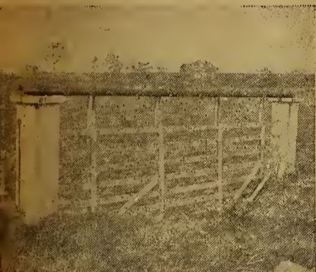
Floodgate anchored to concrete posts
