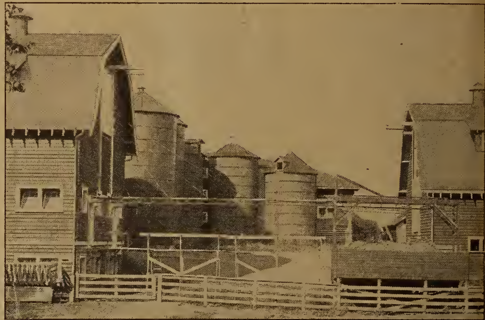
The owner of these buildings believes they have increased the value of his farm more than 50 per cent
