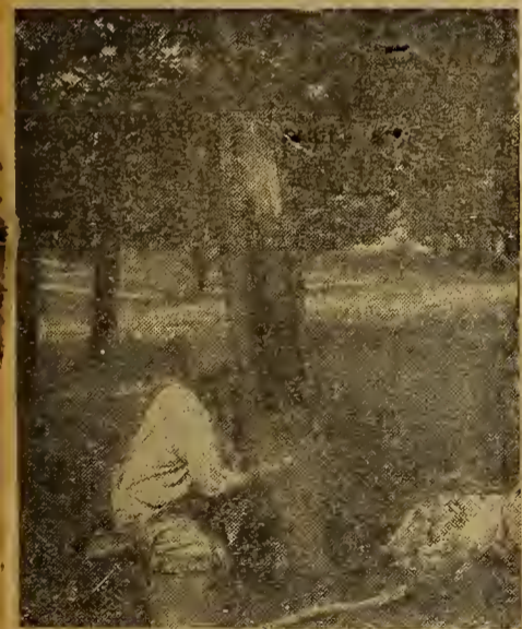
Tree safety by the cement route
