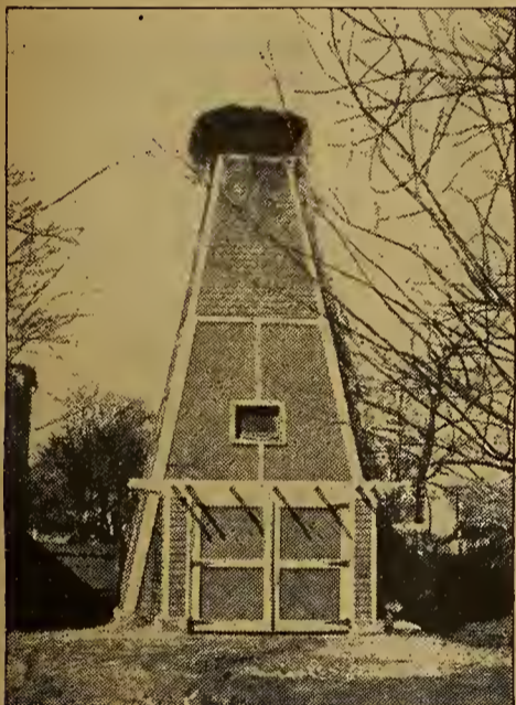
Slight remodeling made this old structure give modern service
