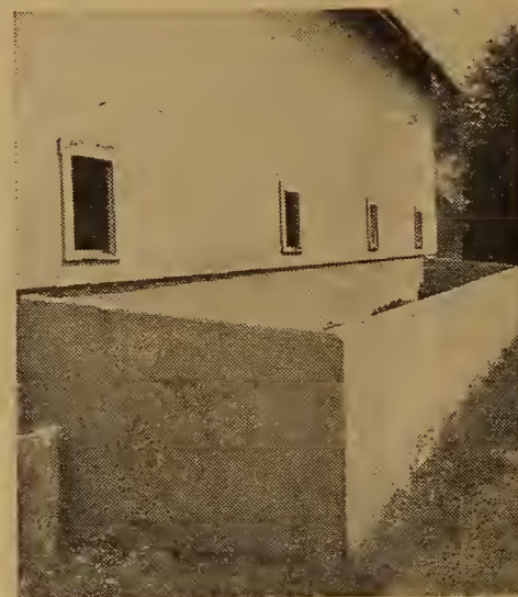
A concrete pit prevents plant food in manure from leaching away
