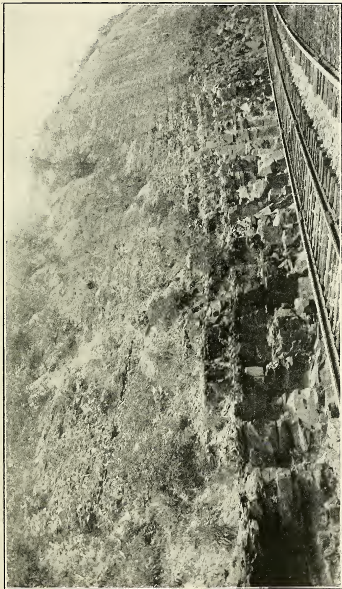
PLATE XV.—Anticline in Hamilton Shales (West End) with Heavy Sandstone Stratum at Base, in deep cut of Baltimore and Ohio Railroad North of North Mountain Station.
